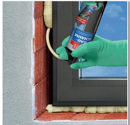
Filling a connection joint on the window.
