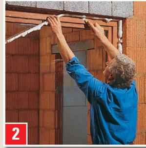
**2** Cut off excessive material with a sharp knife after about 2 hours.
