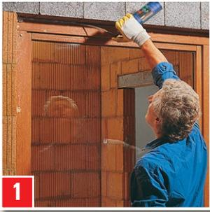
**1** Foaming a window frame: Shake the BAUSCHAUM can well about 20 times. Foam around the window frame.
