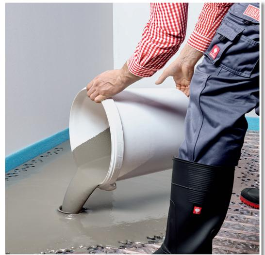
Self-spreading and creates level surfaces on e.g., thin-layered floor warming systems.
