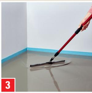
3 Evenly spread the applied mass with a scraper or a rubber slider. Protect the fresh material from draught and sunlight.
