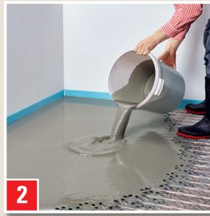
2 Stir bag contents (20 kg) into 4.2 – 4.4L of clean water. Stir again after 3 minutes. Pour out the material section by section and provide sufficient ready mixtures. Apply them one after another at a good pace.
