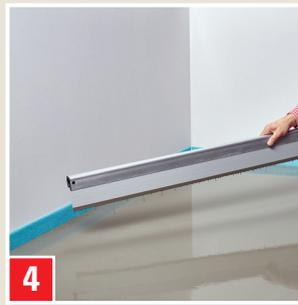
4 The required system covering of 5 mm is measured by dipping an aluminium straight edge and measuring the adhering mortar film. Immediately clean the tool with water.
