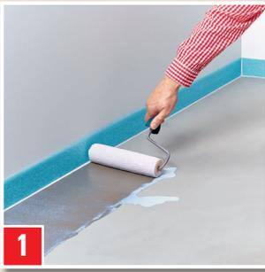
1 Apply BESTE BASIS on the substrate with a paint roller and allow drying for 1 to 4 hours depending on the absorbing capacity.
