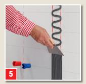
For bonding system installation parts to ABDICHTUNGSBAHN (Fig. 5-7): Apply the BOMBEN-FEST and spread a 12 cm wide layer in the middle over the area of the joint with a toothed trowel.
