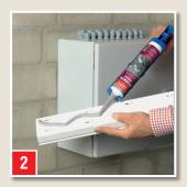
With a sealant gun, apply adhesive to the rear side of the cable duct.
