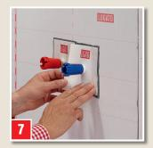
Embed system installation parts (DICHTUNGSMANSCHETTE in this case) in the applied BOMBENFEST adhesive and smooth out.
