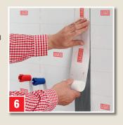
Apply DICHTUNGSBAND in theadhesive. Then smooth out until all creases or bubbles have been removed.
