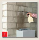
Gluing a cable duct to sand-lime masonry: moistening of absorbent surfaces.
