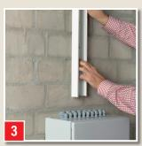
Within 5 minutes, join the components together, press on and align. Press against or support heavy components until hardening.
